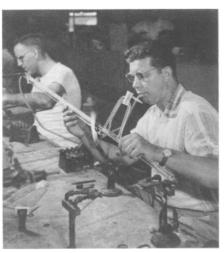
BLOWING HARD GLASS — Intricate laboratory ware, such as this automatic burette, can be produced which will remain accurate over a wide temperature range. Kimax glass-measuring equipment, developed by Kimble Glass Company, is said to be completely interworkable with other hard glass apparatus having the same linear coefficient of expansion.
