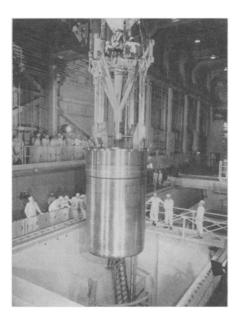
REACTOR'S HEART—This 58-ton nuclear core is being lowered into position in the nation's first full-scale atomic power plant at Shippingport, Pa. When this giant electrical generating station, a product of the Atomic Energy Commission, Westinghouse Electric Corporation and the Duquesne Light Company, goes into operation, the U.S. will come of age in the atomic power era.
