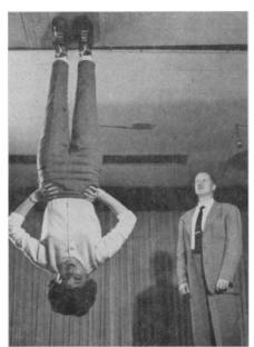
WALKING ON THE CEILING— Nancy Wendler demonstrates shoes for weightless conditions (above). The shoes' developer, John F. Heard, engineer in space technology at Martin Marietta Corporation, Denver, Colo., looks on. Tiny nylon hooks of special Velcro material (right) fastened to the ceiling fit into eyes under the shoes and allow walking on the ceiling.
