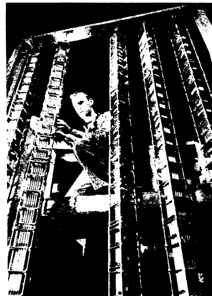
CHECKING FUEL BUNDLES— Atomic power technician, Lester Race, checks fuel bundles for Yankee Electric Company's nuclear plant whose reactor was built by Westinghouse Electric Corporation, Pittsburgh, Pa.
