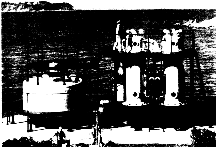
WATER CONVERTER —Model shows how pilot plant to be built by General Electric Company, Schenectady, N.Y., will look when constructed at U.S. Office of Saline Water's new test facility, Wrightsville Beach, N.C. Purpose of the plant is to explore large-scale conversion of sea and brackish water.
