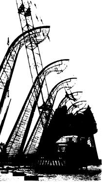
GIANT STEEL SERPENTS-The world's largest truck crane is being used to erect the steel skeletons for the ultramodern columns of the Dulles International Air Terminal building. These steel skeletons will be encased in concrete. From the columns a cable-hung roof will be suspended. To pour concrete for the curved columns, which lean outward to resist the pull of the cabled roof, forms of glass-fiber sheets and plywood are used,
