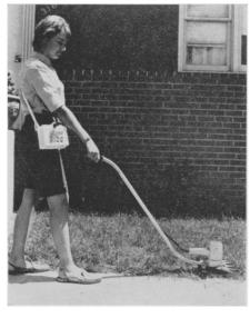
POWER GRASS SHEARS, shown in photograph, simplify lawn trimming and run on a 12-volt rechargeable battery carried by a strap from the shoulders. No long-trailing electric cord from a 115-volt house current is necessary, thus eliminating risk of dangerous shock even if the cord from the motor to the battery should be accidentally cut. The shears can be detached for use on close-up hand-trimming chores.
