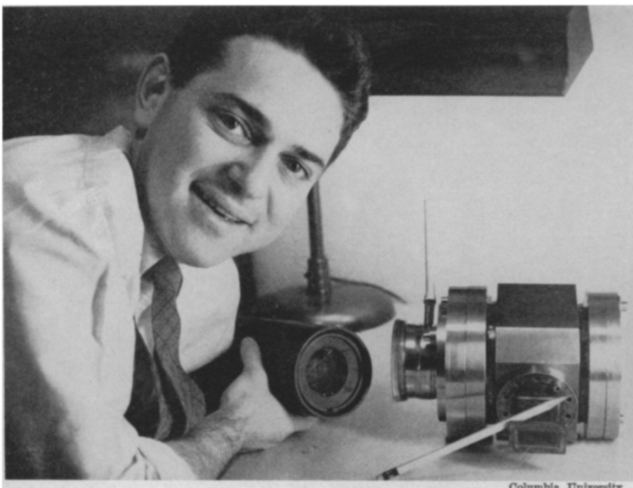
MOST ACCURATE TIME —Dr. Paul Davidovits holds the rubidium type maser, or atomic clock, he developed at Columbia University's Radiation Laboratory. The instrument can be used to make extremely accurate measurement of time and distance from satellites or high-flying airplanes.
