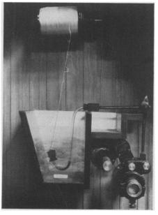
THREADS OF ARTIFICIAL SILK Are made by this model which is on exhibit in the U. S. National Museum. It differs from a commercial machine only in having one spinneret instead of many
