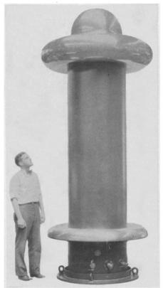
NEW WEAPON AGAINST CANCER Seven hundred thousand volts will be made easily available to the California Institute of Technology scientists by two new giant X-ray transformers made by engineers of the General Electric Company. One of these, shown above, has already been shipped to the coast and the other is nearing completion.
