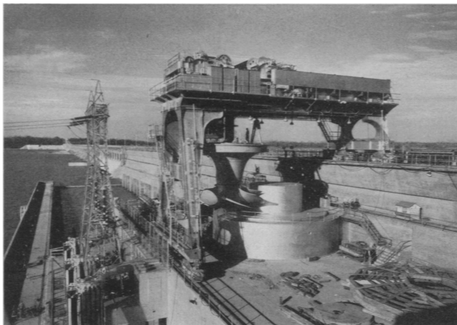
GIANT HOISTING CRANE
