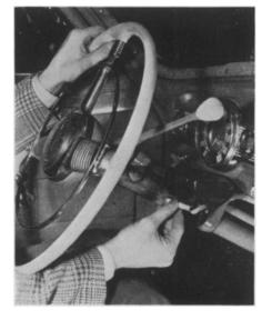
CIGARETTE DISPENSER and lighter, for use in an automobile as shown in the picture, drops a single cigarette into a small trough with a single pressure on a lever. In the trough, it is held by a spring against a hot filament and in four seconds is lighted.
