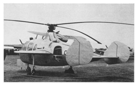
RESEMBLES AIRPLANE—This British experimental helicopter looks like orthodox aircraft because it has a normal tail with twin rudders and stub wings. Advantages claimed for its unique design are greater safety, higher forward speed and greater comfort. It can seat four people including the pilot.
