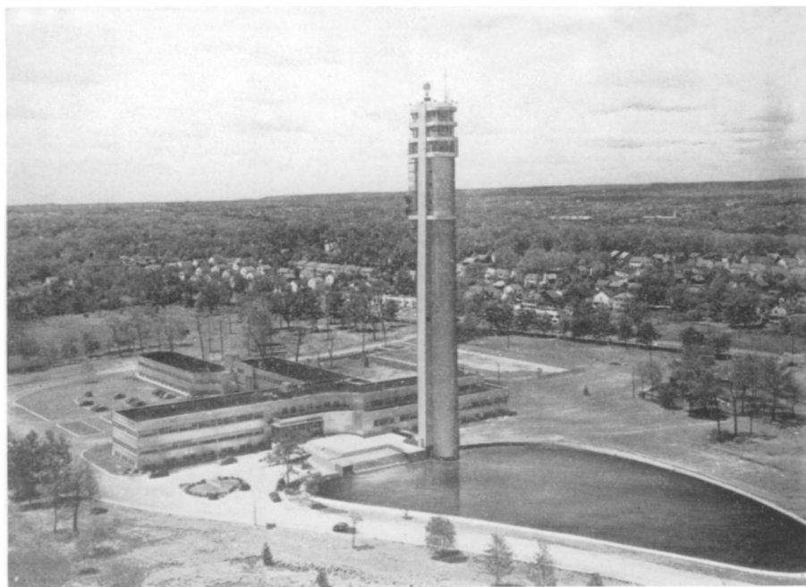
TWO-COLOR RADAR —One of the projects being experimented with in this microwave laboratory tower at Nutley, N. J.
