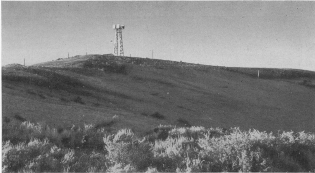
Radio-relay station at Evanston, Wyoming
