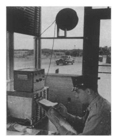
RADAR WARNING - From the round reflector in the window, a beam of short radio waves is aimed down the road. The approaching automobile sends back an echo that causes a warning bell to ring inside the guard house, calling the attention of the guard to the arrival of a visitor or intruder.
