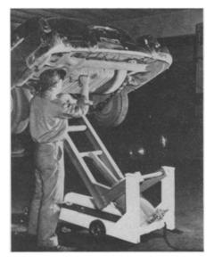
automatic safety lock holds the lift at any of its ten working heights, one of which is shown in the photograph.
