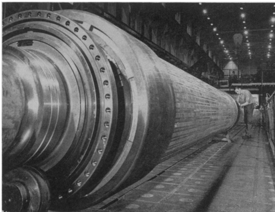
HIGHEST STEAM TEMPERATURE —This generator rotor will be turned by a turbine that operates with the highest steam temperatures ever used for this purpose. Thirty-two feet long and weighing 100,000 pounds, General Electric reports it will operate at 1,100 degrees Fahrenheit.
