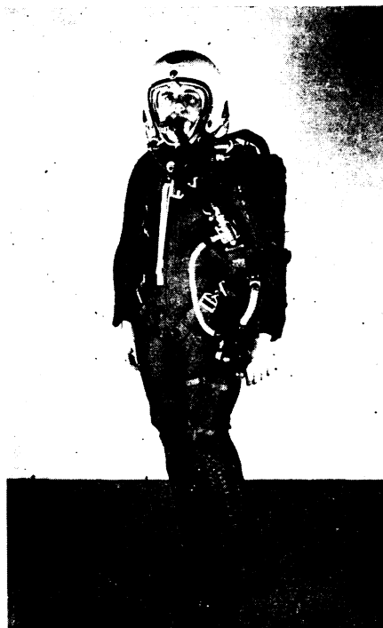
EMERGENCY FLYING SUIT —The new United States high altitude pressure suit, the T-1, being tested by a pilot at the Aeromedical Laboratory, Wright Air Development Center, Dayton, Ohio, will enable pilots to survive in the near vacuum of the upper atmosphere.
