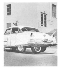
cars. The car is nosed into a parking space and a dashboard lever is turned. The spare tire lowers hydraulically until it lifts the car's rear wheels as shown in the photograph, then it rolls the rear end of the car to the curb. The device also can be used to get the car out of a tight spot.
