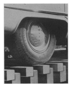
into the parking shelf and are set down. The movable elevator floor is made of parallel beams that slip between smaller beams of the parking shelf.
