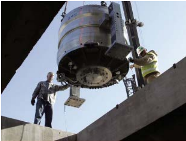
FAVORABLE SPIN — Engineers lower a flywheel prototype into a concrete bunker for a safe test at high speeds.
