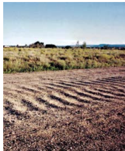
TROUBLED TRAVEL Vehicles passing constantly over dirt roads create an irksome washboard surface, seen here on a road in Australia.
