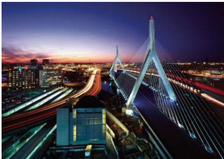
CHARISMATIC CABLES — Eye-catching cable-stayed bridges, like Boston’s Zakim-Bunker Hill Bridge, are becoming city showpieces.
