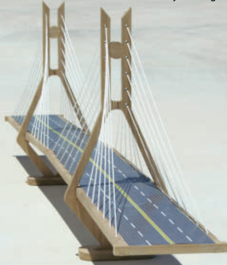
The Cable-Stayed Bridge
