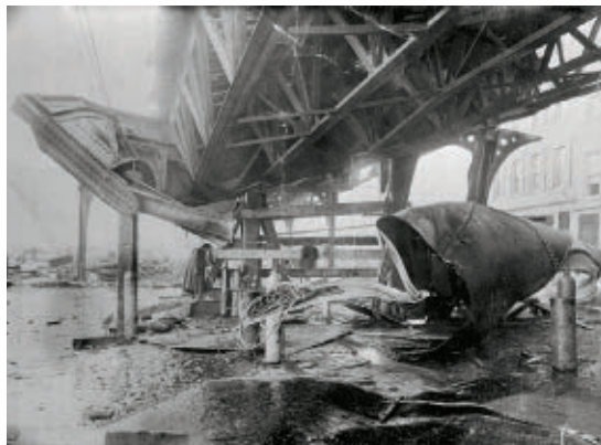
Boston's Great Molasses Flood probably began with a cracked tank. In 1919, more than 8 million liters of goo rushed through city streets, twisting structures (train track, shown) and causing 21 deaths.
