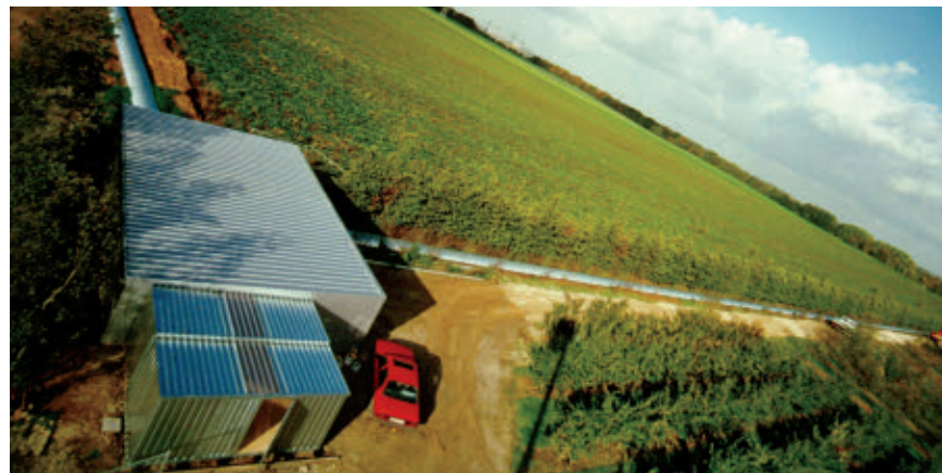
The GEO600 experiment in Germany may be able to detect a jitter in spacetime by picking up sideways motion in a beam splitter that divides one laser beam into two. The beams then travel down perpendicular arms (shown) 600 meters long.
