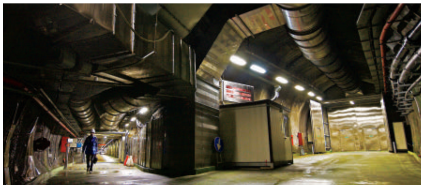
The two tunnels at the entrance of the underground Gran Sasso Laboratory in Italy, where the XENON100, CRESST and DAMA experiments are housed.
