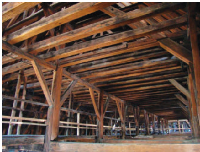
The “forest” of Notre Dame held up the cathedral’s roof and spire. It was destroyed in the fire, but researchers hope to study the charred remains of the medieval oak beams to learn about climate change.
