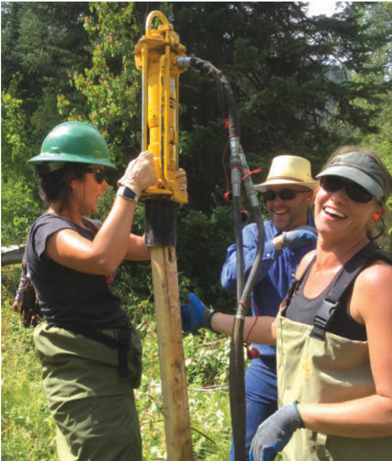
Staff from the USDA Natural Resources Conservation Service pound posts to build a beaver dam analog across Birch Creek in Idaho in 2016. The effort gave nine relocated beavers a head start to create their own dam complexes.
