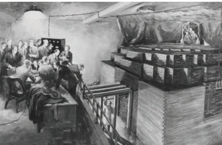
The first controlled, self-sustaining nuclear chain reaction took place in a pile of uranium and graphite (at right in this illustration) at the University of Chicago in 1942.
