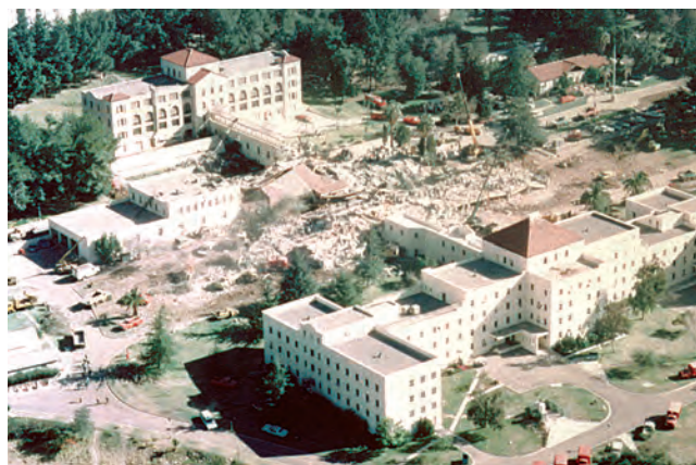
FATAL FAILURE — Two Veterans Administration hospital buildings were reduced to rubble during the San Fernando, Calif., earthquake of 1971, causing the death of 46 people.
