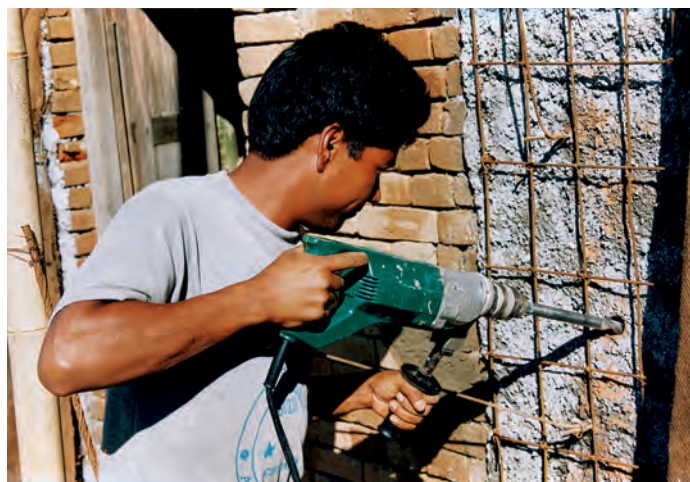
SUBTLE STRENGTH — The exposed steel grid is a simple form of seismic bracing. Fitted by local masons, the mesh should keep this school in Nepal standing during and after a quake.
