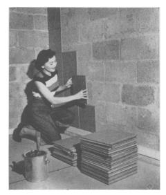
WONDERWALL, TWO IN ONE— The new Velon plastic wall panel not only insulates but decorates. Being applied directly over cinder block walls in the above picture, it can also be installed on wood, plaster, brick or concrete. The tongued and grooved edges make perfect fit and alignment
