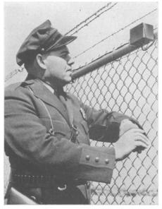
The guard in the picture is reporting "All's Well" to a central guard station in one of our war factories, protected by an acoustic fence. This fence is all ears. If tampered with anywhere, sounds are heard at the central station and an annunciator indicates where the disturbance took place. Even a dog crawling under the fence sets off the alarm. Although the guard in the picture is a message from any point along the fence by tapping it out in code.
