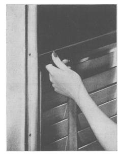
THE PLASTIC STRIP seen on the left side of the picture prevents light from leaking around the edge of a blackout shade. The molding is easily attached to any window frame by means of screws.
