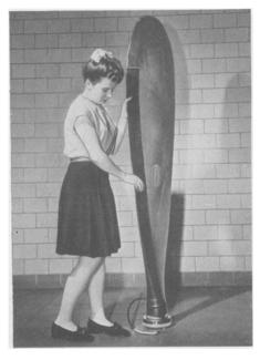
ing of electricity-conducting rubber between two sheets of non-conducting rubber. Passage of electricity through the center sheet causes heat. Ice guard section of the blade is being held in the picture. Science News Letter, April 19, 1947
