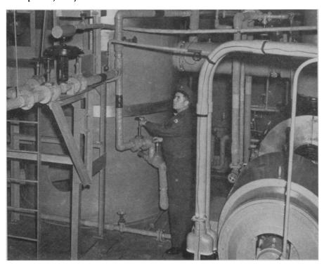
FRESH WATER FROM SALT—Ocean water is changed to fresh water in this huge distillation plant, developed and tested by the Corps of Engineers at Boston Army Base and now operated at Kindley (U.S.) Air Force Base in Bermuda. Drinking water produced by this plant costs ten times what U.S. communities pay for natural fresh water, but in Bermuda, no water is available from rivers or wells. Natives must catch rain water in containers on the roof-tops of their homes.
