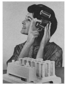
ELECTRIC HAIR CURLER allows hair to be set quickly at the home dressing table. The compact unit can be plugged into the household current and consists of a set of insert tubes that fit in the device for heating and a supply of cordless rollers. The electric unit, thermostatically controlled, heats the tubes for insertion in the rollers previously arranged on the head.
