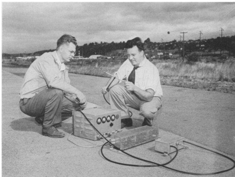
**MEASURING SPEED OF FAST PLANES**—This is the equipment used in the plane with the improved Doppler system of measuring speed. It receives a radio beam from a ground station, doubles its frequency, and returns it to the ground.
